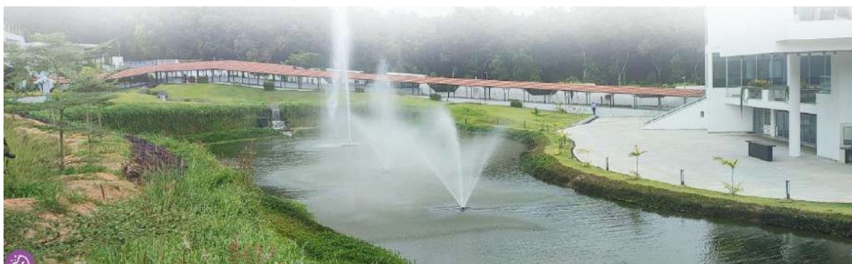
Figure 2.1 – Rainwater harvesting at our Trivandrum Campus
